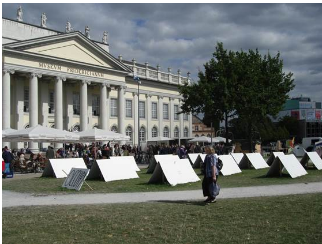
3.24. picture: Dokumenta 2012 – the main exhibition building, Fridericianum with protesters' tents, Kassel, Germany. (Photo: Andrea Kárpáti)
