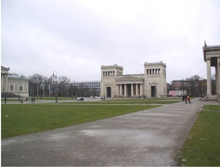
5.4. picture: The Königsplatz (King's Square) in Munich, Germany, with three museum buildings erected in the style of ancient Greece. On the right: façade of the Glyptothek, dedicated to classic Greek and Roman sculpture. It can only be approached through the square – a spatial experience that prepares for the visit. (Photo: Tamás Vásárhelyi)
